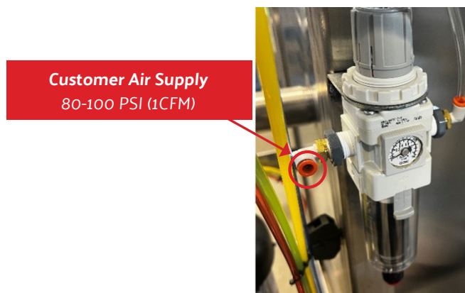
fig. 4 - 1 - Air regulator supply line
