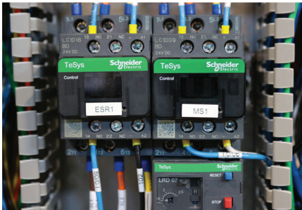
Fig. 3.3 - 6 - MS1 contact location
