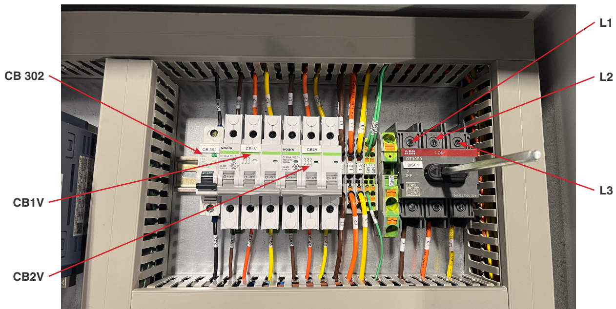
Fig. 3.3 - 1 - Customer 3PH connection
