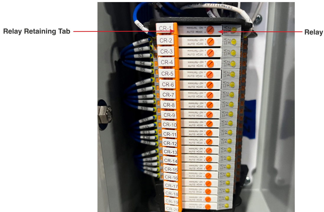
Fig. 7.6 - 1 - Relay replacement
